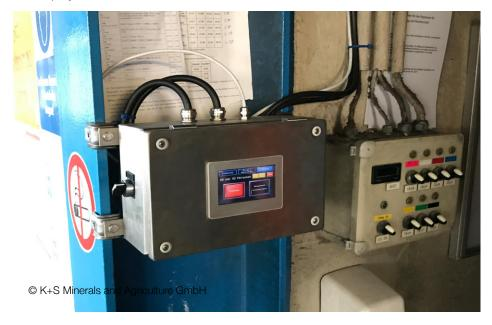
In addition to the different shifts, malfunctions or other messages can also be shown on the display. In accordance with the requirements in the mine - darkness, crude salts, dust exposure - the LED system impresses with luminous as well as high-contrast, yet fanless and maintenance-free technology. The robust "packaging" in a stainless steel housing completes the picture.
